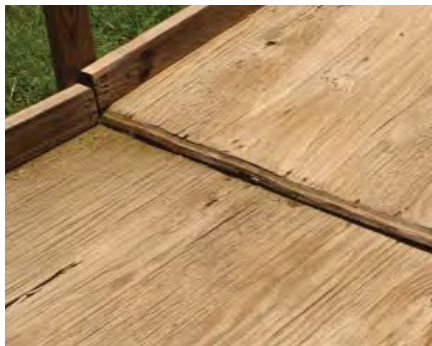
Uneven, bumpy transitions, warped slick surface.
